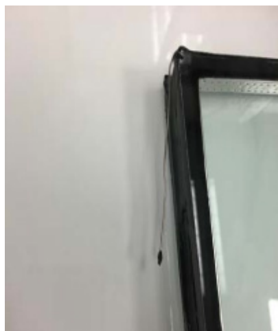
Figure 2: Apply silicone dab to tube end
