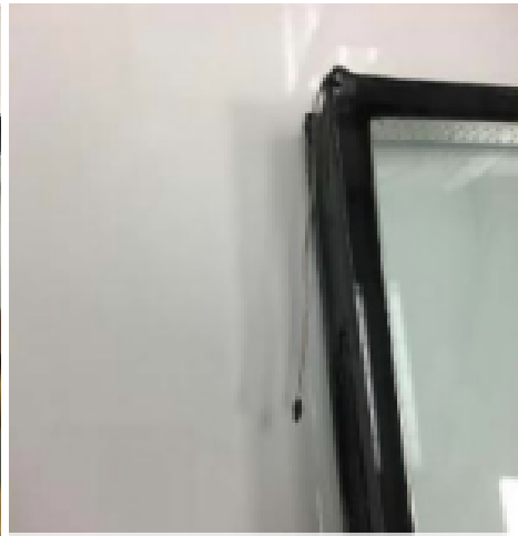
Figure 2: Apply silicone dab to tube end
